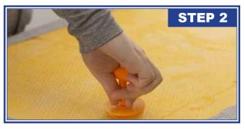
See <u>Appendix A</u> for suggested Rotofast install locations based on your panel size. Screw Rotofast Snap-On Anchors into the back of the panel using the Hex tool. Do not over-tighten.
