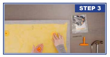
Insert marking plugs into the Snap-On Anchors.
