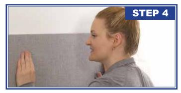
Push the panel against the surface to mark anchor locations.
