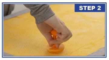
See <u>Appendix A</u> for suggested Rotofast install locations based on your panel size. Screw Rotofast Snap-On Anchors into the back of the panel using the Hex tool. Do not over-tighten.
