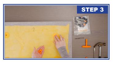
Insert marking plugs into the Snap-On Anchors.
