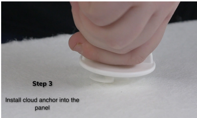
Install cloud anchor into the cut
