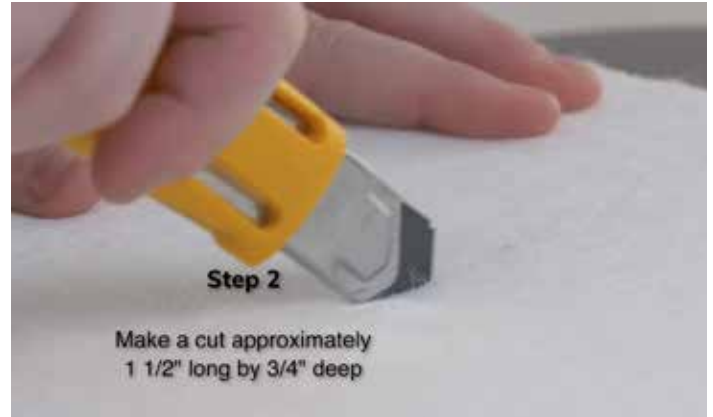
Cut polyester with a sharp utility knife
